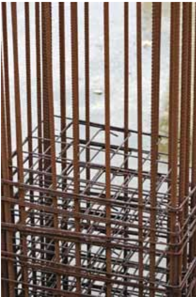
Steel reinforcing bars
