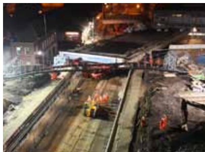
Caversham Road Bridge 13
