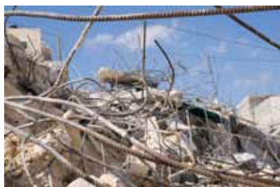
Reinforcing steel in a demolished building
