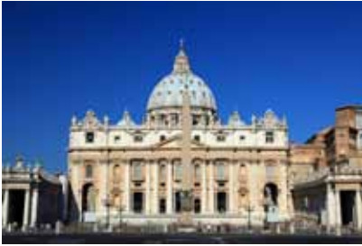
St Peter's Basilica in Rome was built using reclaimed blocks from the Colosseum
