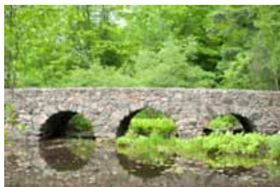
A masonry footbridge
