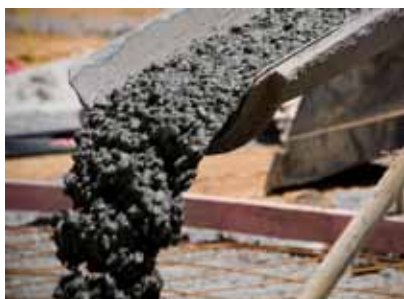
Pouring reinforced concrete
