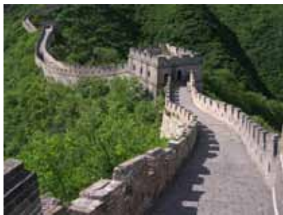
The Great Wall of China
