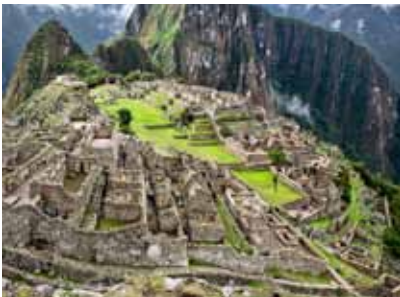
A few old masonry walls at Machu Picchu
