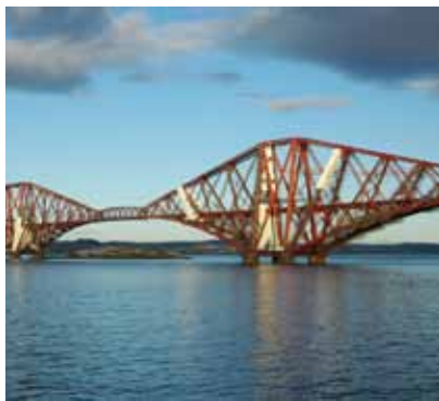
The well-painted Forth Road bridge
