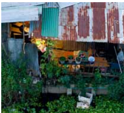
Inventive reuse of steel
