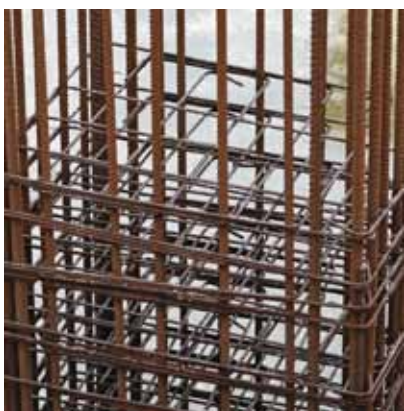
Steel reinforcing bars, used to provide strength and stiffness in tension in concrete structures
